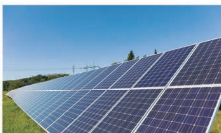
Yuzhou Peak Photovoltaic Power Station Project
